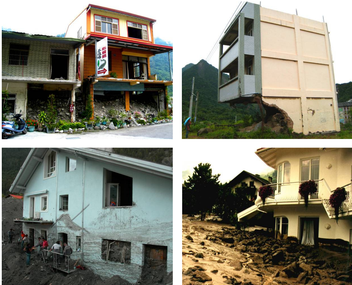
Fig. 4 Typical damage patterns for buildings affected by torrent processes in Taiwan (top) and Austria (bottom). Upper left: Songhe community, Taiwan, event of August 2004, upper right: Min-Zu community, Taiwan, event of August 2009, lower left: Pfunds community, Austria, event of August 2005, lower right: Wartschensiedlung village, event of August 1997. Credits: upper left: S. Fuchs (27 August 2011), upper right: S. Fuchs (28 August 2011), lower left: Gebietsbauleitung 6.2 (23 August 2005), lower right: anonymous (event of 16 August 1997).
